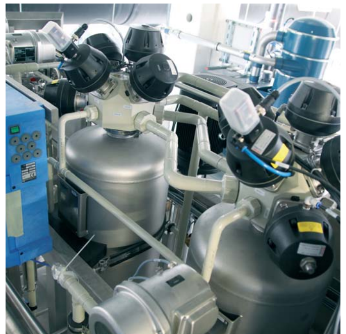
Ion exchanger - compact design with multi-port valve blocks
